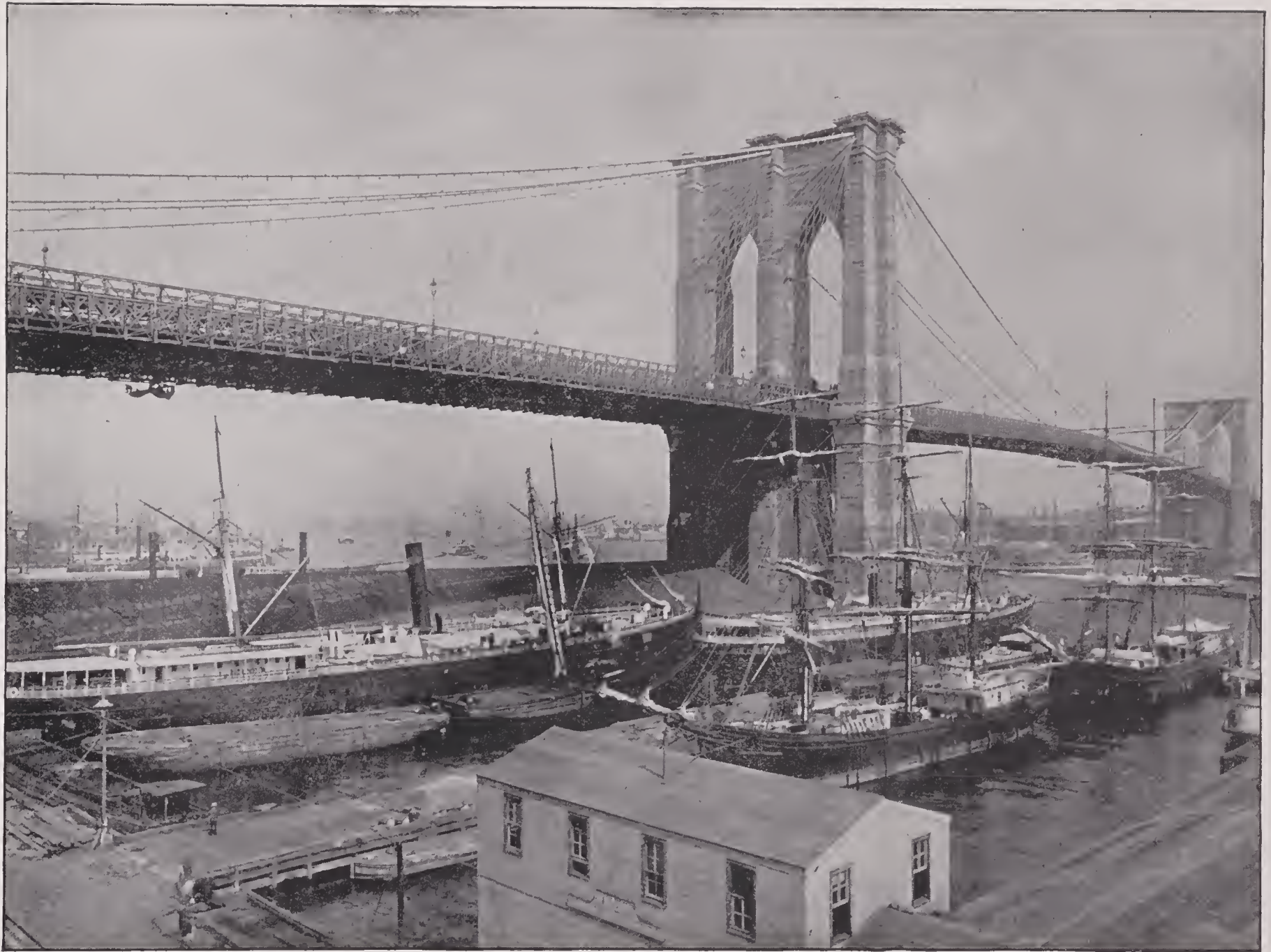
BROOKLYN BRIDGE, NEW YORK CITY, N. Y. —This bridge, connecting New York with Brooklyn, is by far the largest suspension bridge yet constructed. The work was commenced in 1870, and opened for traffic on May 24, 1883. The central span, from tower to tower, measures fifteen hundred and ninety-five and one-half feet. In the centre is a foot-way, fifteen and one-half feet wide, and raised twelve feet above the other passages, affording an open view on both sides. There are tracks on each side for cable cars, worked by a stationary engine on the Brooklyn side, and on the outside are wagon-ways. The entire cost was $15,500,000.
